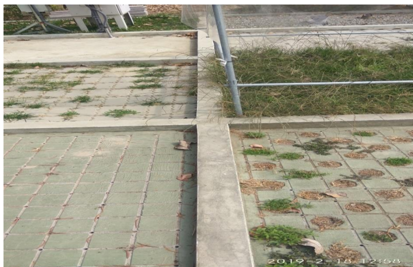
Fig(c) permeable pavement cell
